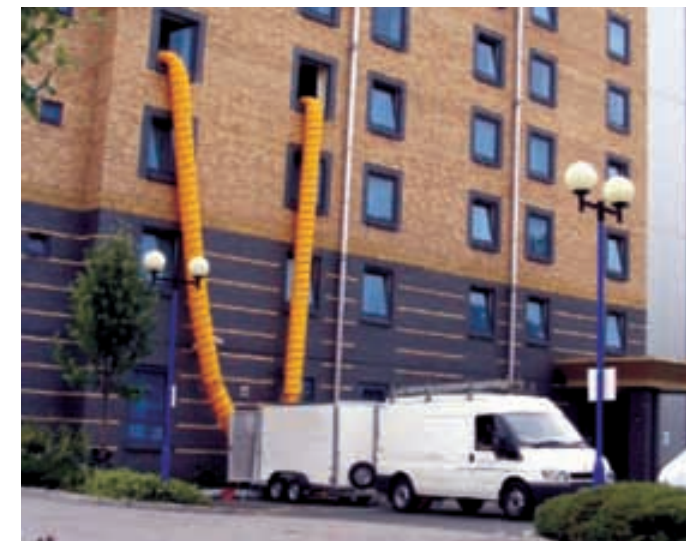
Hot air generated by the diesel heater unit is ducted into hotel rooms
