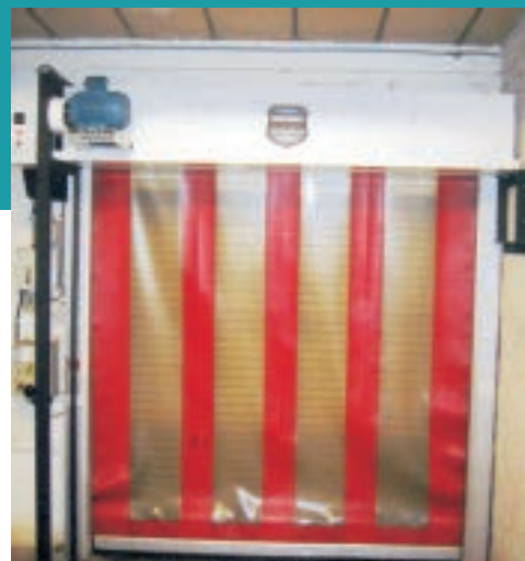
The fitted Enershield DSH-120 air barrier over the existing rapid-roll door
