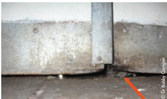
The author took this photo one night as mice were coming and going from beneath a delivery door to a food store. Notice the approaching mouse (see arrow) and heavy mouse smears at the base of the right door. Pest proofing is a scientific sub-discipline and trade of urban rodentology. Most property owners (and even many maintenance staff) have incomplete knowledge about how to properly pest-proof doors, repair holes, cap off block walls and the like
