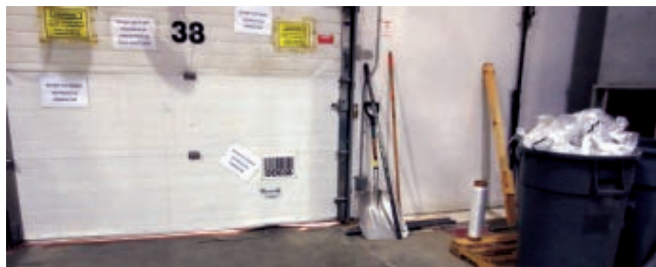
A typical overhead warehouse door. Note the poor door sealing at the base and the overlooked rope-pull causing a gap. Essentially, any exterior light seen from the inside is usually likely to permit rodent entry
