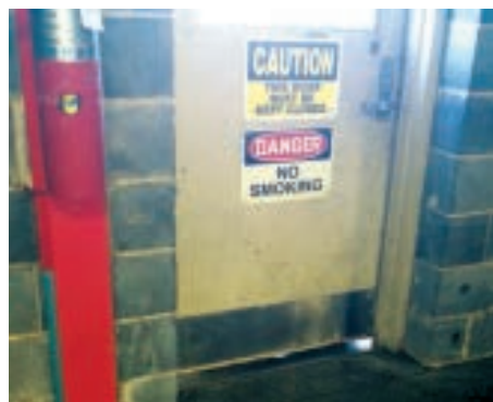
A typical single-swing door. The sign says one thing; the gap, bottom right, another
