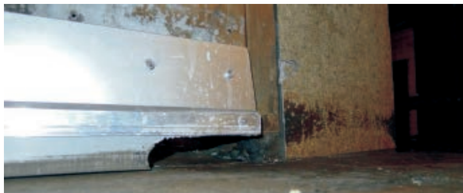
The grey vinyl strip on the base of this door is a weather strip. Note how the rodents were able to easily gnaw through it (also note the tooth marks in the vinyl)
