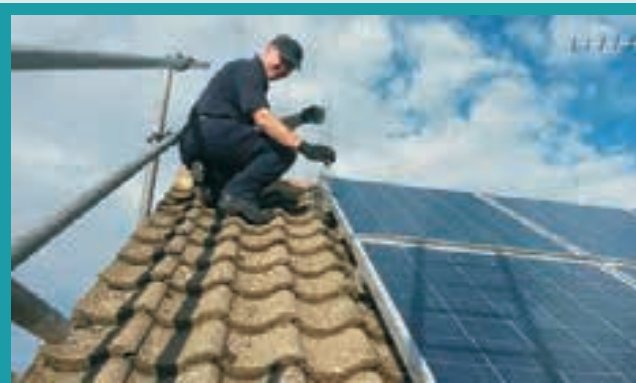
Above: Martin Gill of MG Pest Control attaches the mesh to the solar panels Right: pigeon guano, nest debris and the like that can soon block gutters etc
