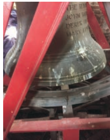
Acidic bird droppings were damaging the bells
