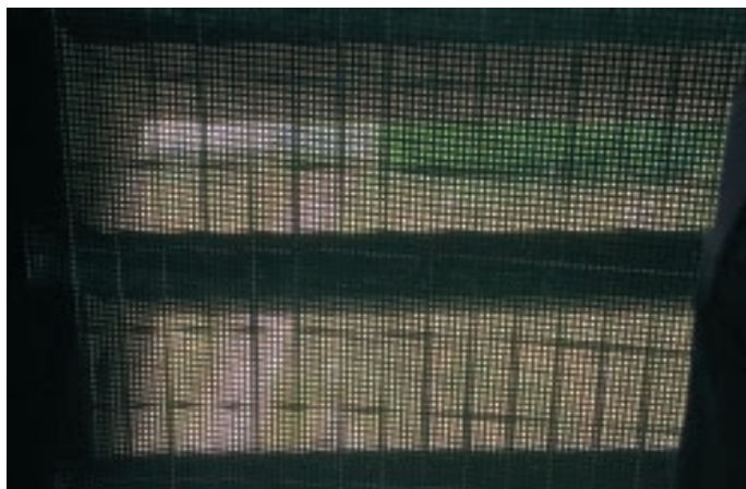
Small gauge, galvanized weld mesh was fitted to prevent re-entry
