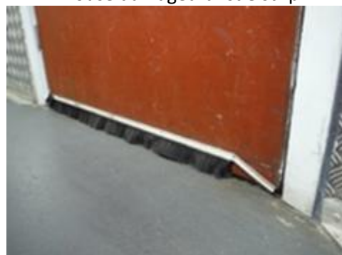
Carrier on brush strip is damaged and not been adequately crimped; bristles have fallen out
