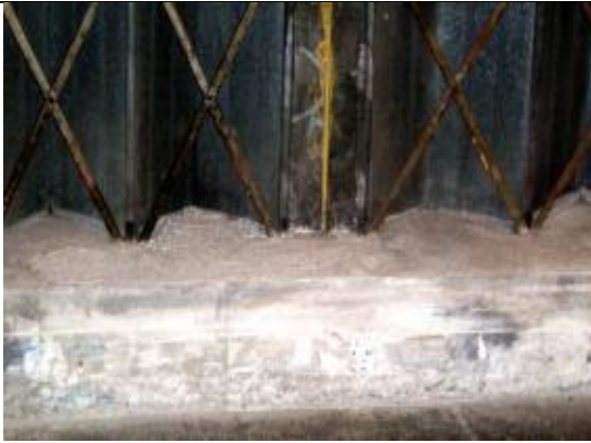
Base of redundant concertina door embedded in concrete (a triangular fillet of cement would also serve, and can be easily removed if needed)
