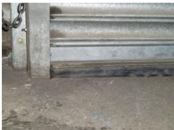
Roller door compression seal fitting tightly to floor and doorframe
