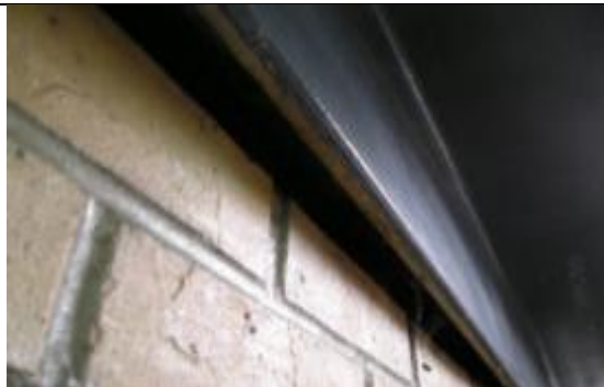
Gap between cladding and brick wall
