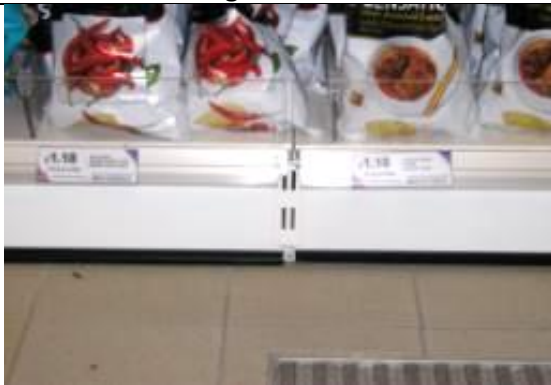
Kick plate in good condition and easily removable for inspection
