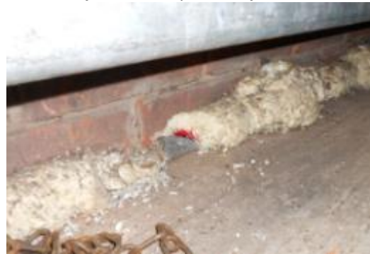
Excessive use of expanding foam to seal a wall-floor junction. Mice have penetrated this
