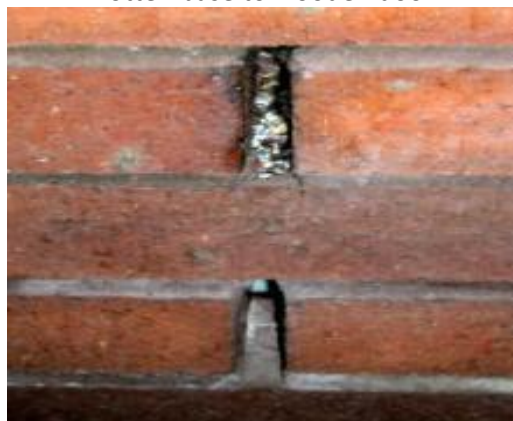
Weep (ventilation) holes with smears, where mice are using them to access the wall cavity
