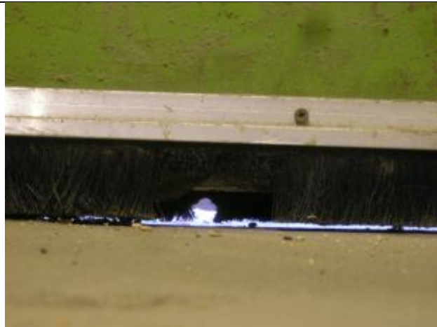
Mouse damaged bristle strip
