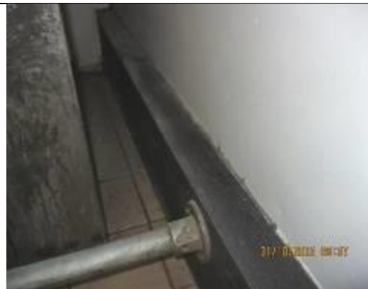
Hollow box sections along the wall-floor junction
