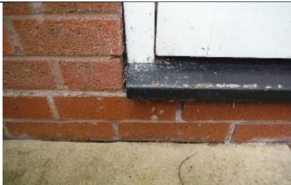
Door frame in good condition
