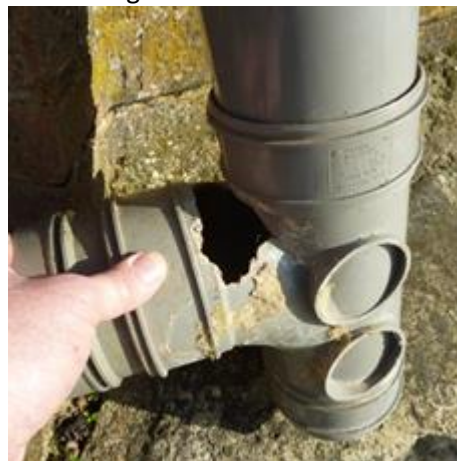
Rat damage to plastic foul-water drainage pipework
