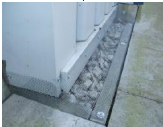
Mesh proofing around base of cladding panels; expensive and unlikely to be effective
