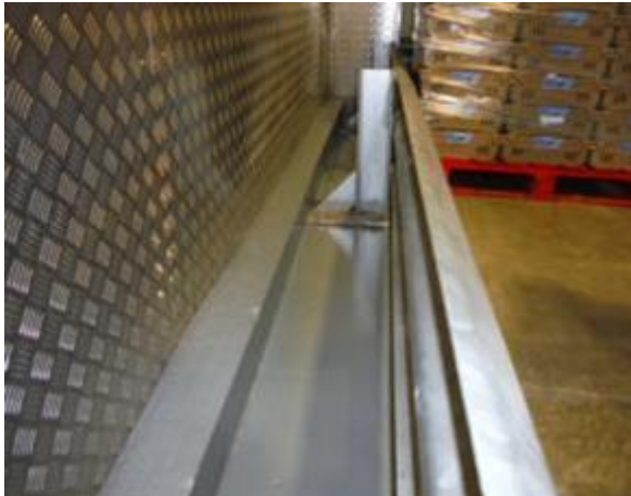
Chilled warehouse with protection barriers and wall-floor junction which cannot be penetrated by rodents
