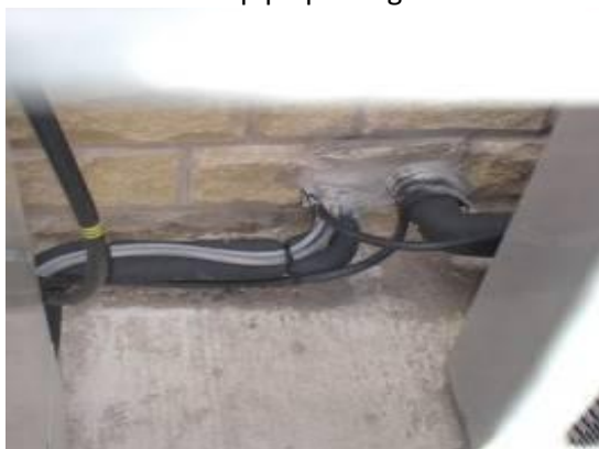
Sealed pipes passing through wall
