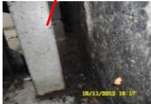
Gaps and voids in external walls provide harbourage areas for pest
