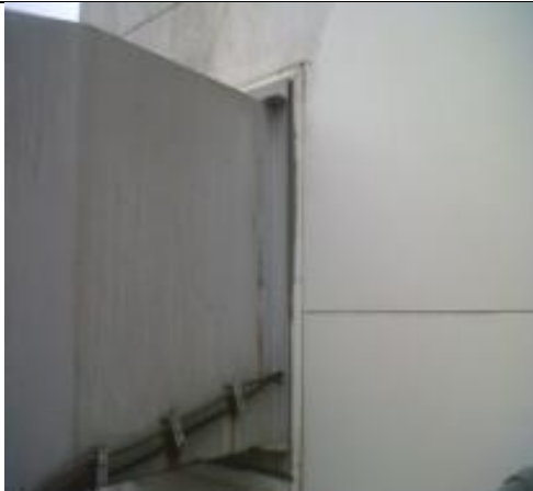
Compactor chute, well sealed to the outside of the building
