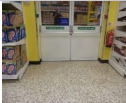
Panels either side of doorway have a small void between them and the blockwork wall, but no access to this is possible.
