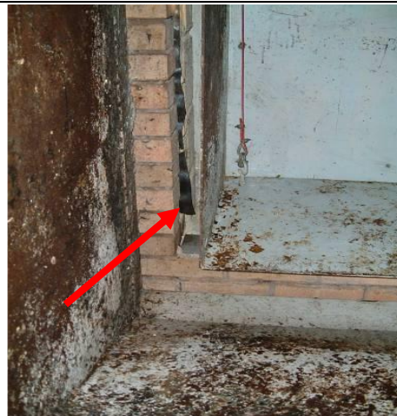
Inadequate seal between compactor chute and cavity wall
