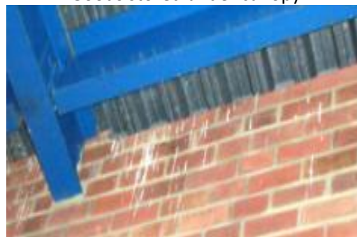
Gap between wall and roof colonised by sparrows
