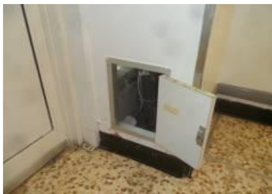
Hinged inspection panel
