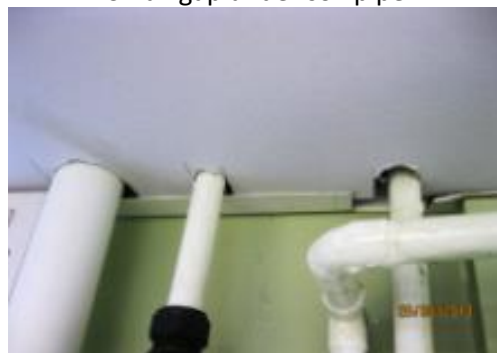
Gaps around services passing into false ceiling
