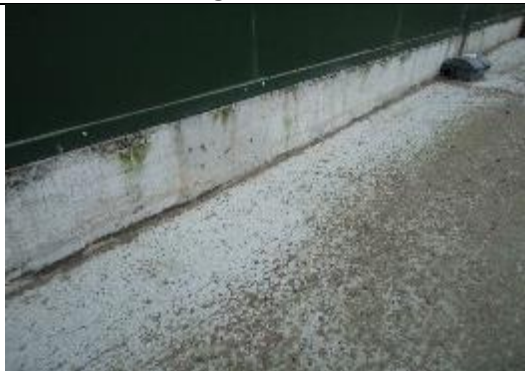
Solid concrete joint between wall base and floor
