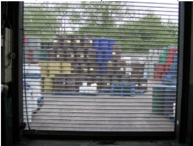
A 'ventilated' roller door allows airflow but denies entry to flying insects and birds
