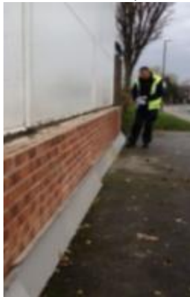
Joint between cladding panels and wall being sealed
