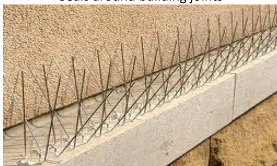
Wall ledges fitted with bird spikes
