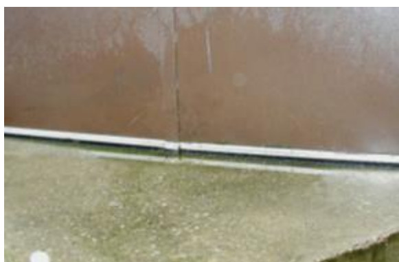
Bristle strip fitted to effect a tight seal
