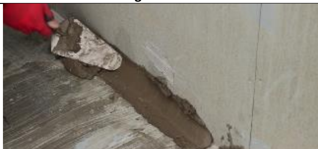
Installing a triangular fillet of cement around the wall-floor junction
