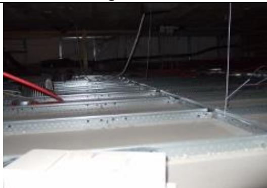
Ceiling void is clear and easily inspected
