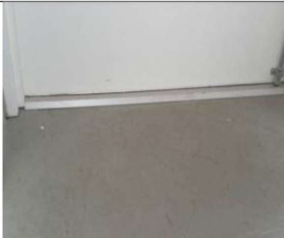
Close fitting door; no additional seal required
