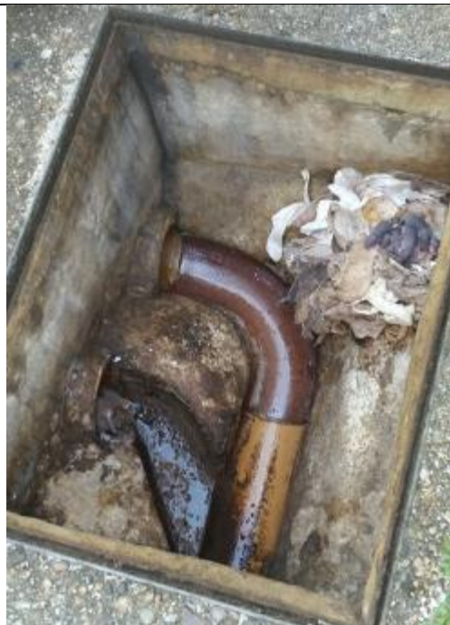
A rat nest in the sewer system
