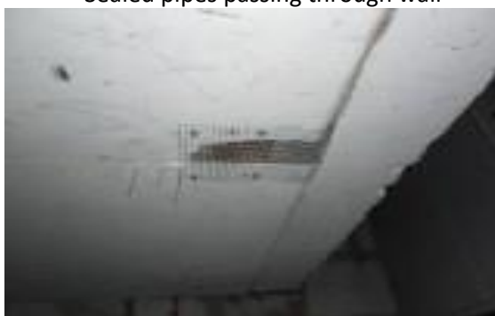
Ceiling hole sealed with wire mesh
