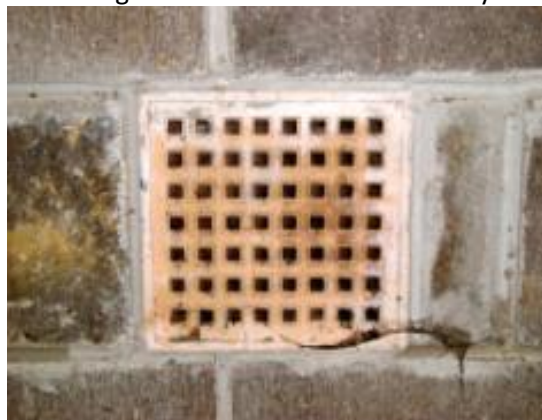
Unproofed airbrick; holes are large enough for mice to enter
