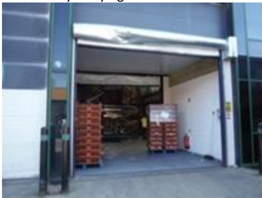
An airlock, with inner and outer rapid roll doors. It would, of course, be better if at least one of these was kept closed at all times!
