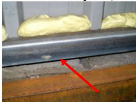
Foam 'proofing' between cladding and supporting metalwork, but leaving the wall cavity still open (arrowed)
