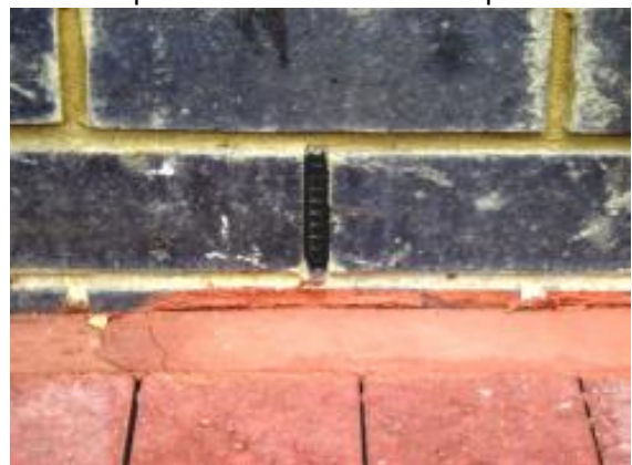
Weep (ventilation) hole proofed with ventilated plastic plugs
