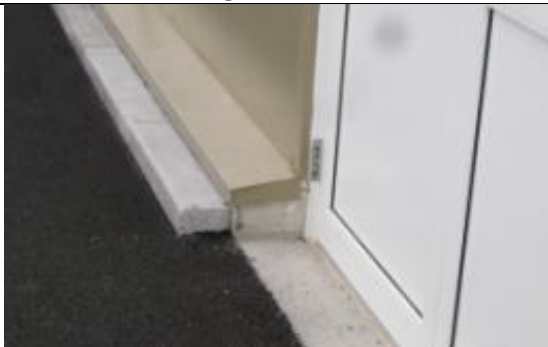
Well-sealed rain-sill
