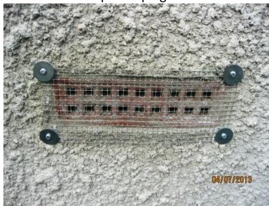
Airbrick fitted with wire mesh cover
