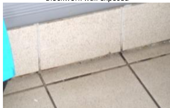
Ceramic tiling with grouting gaps along the base and top of the upstand tiles
