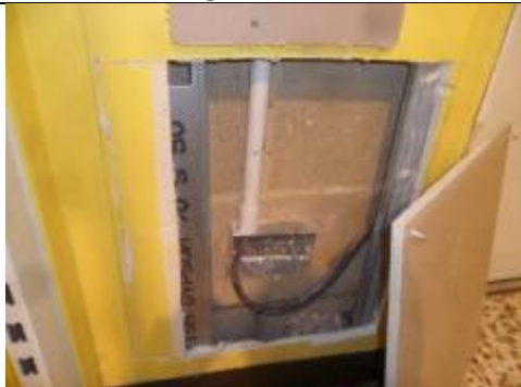
Same wall as in photo shown right, but with an access panel installed
