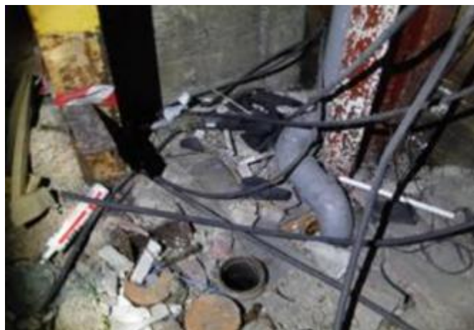
Rubbish, and an uncapped pipe, left in a wall void following construction works
