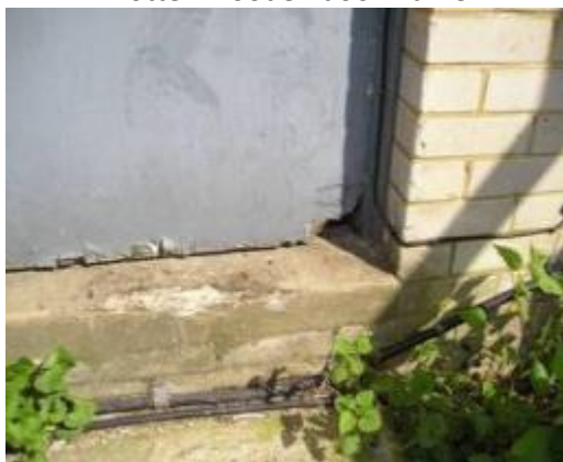
Rotten base to wooden door
