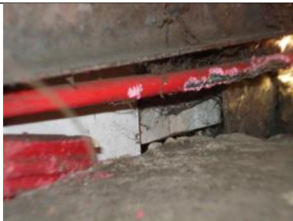
Rodent damage to cabling on a warehouse wall ledge
