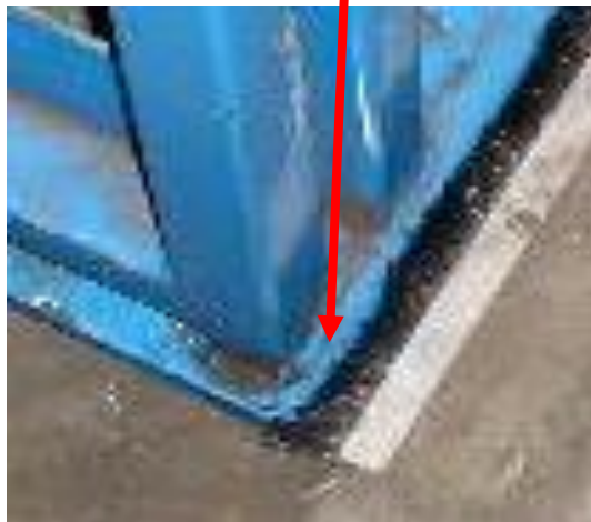
Proofing of a dock leveller with bristle strip
