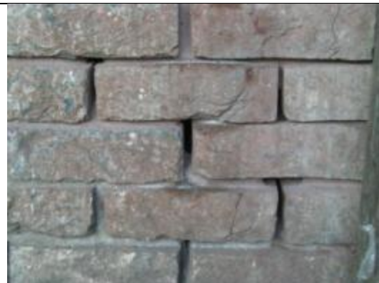
Pointing excavated by mice
