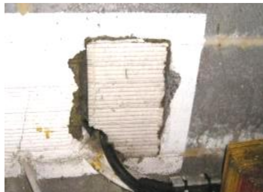
Cables passing through a section of fire retardant insulation; proofing non-existent
