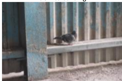
Internal structure un-protected against bird perching
