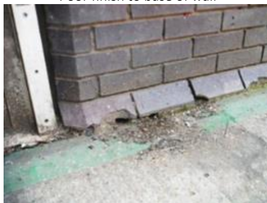
Mouse excavation of wall base; wall cavity has probably been accessed
