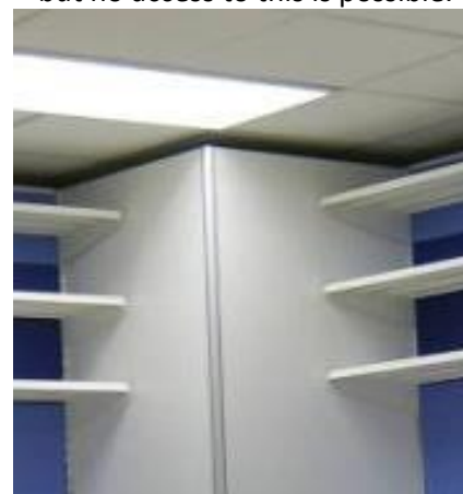
Box section with no access panel
