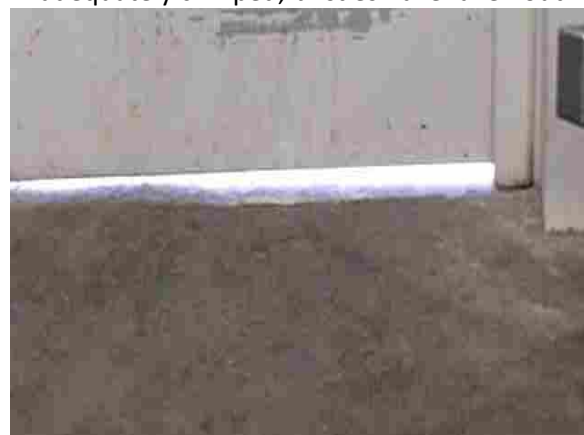
Gap under door with no bristle strip fitted
