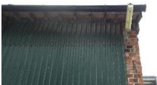
Roof overhang netted off to prevent birds nesting on the roof purlins
