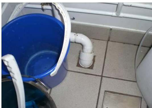
Well-sealed pipe passing into floor
