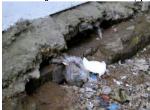
Poor finish to base of wall
