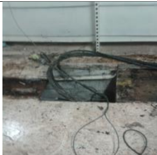
Unsealed holes left under relocated units
