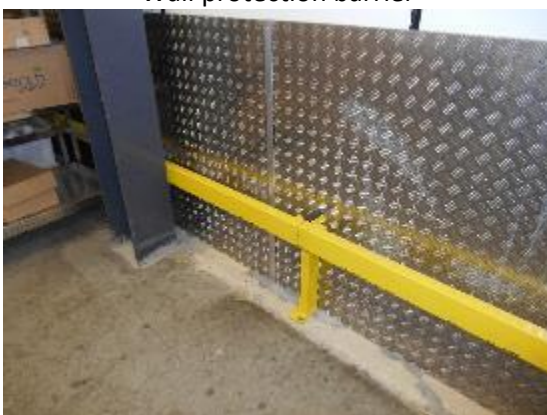
Internal wall protected by well fitted chequer plate
