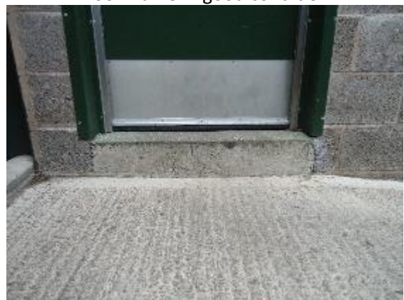
Steel plated door with brush strip fitted
