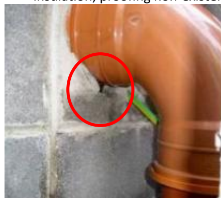
Small gap under soil pipe
