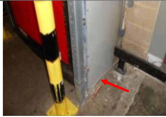
Gap at base of rapid roll door reveal
