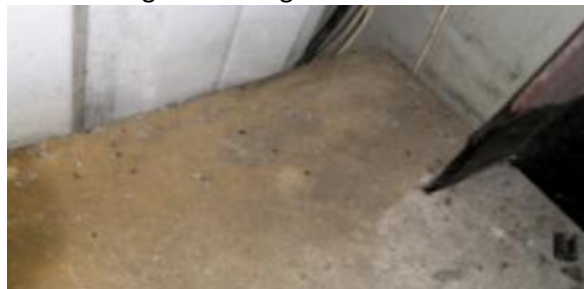
Gaps between external cladding and top of wall ledge.
