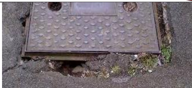
Rat emergence hole around manhole
