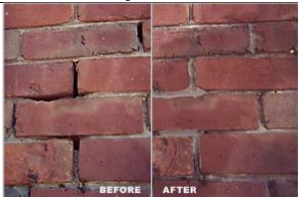
Good pointing work on an older wall
