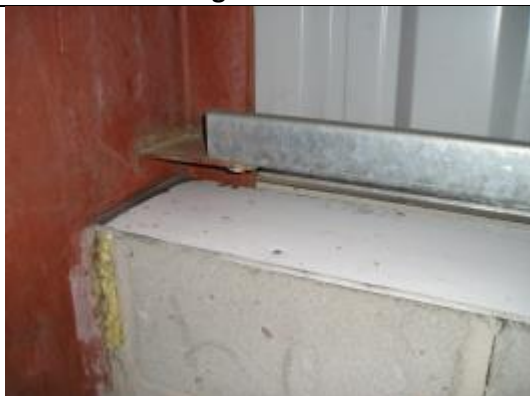
Metal plate used to proof top of block-work cavity wall, with small gaps to RSJ sealed with silicone
