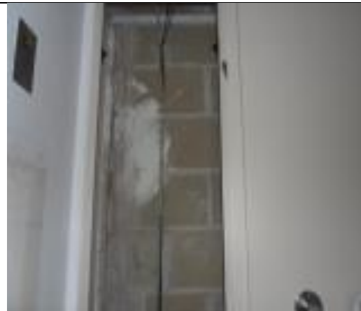
Blockwork wall exposed
