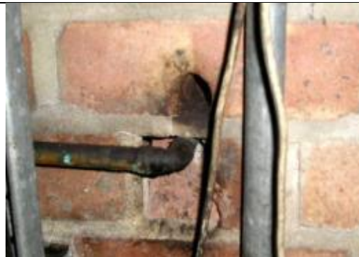
Mouse smeared hole where a pipe has been removed and hole has not been filled
