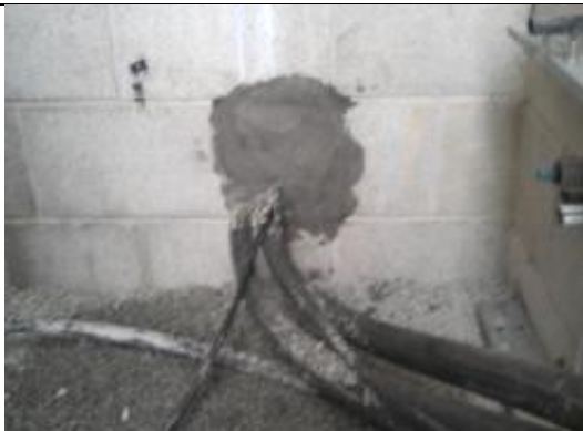
Gaps well sealed with concrete
