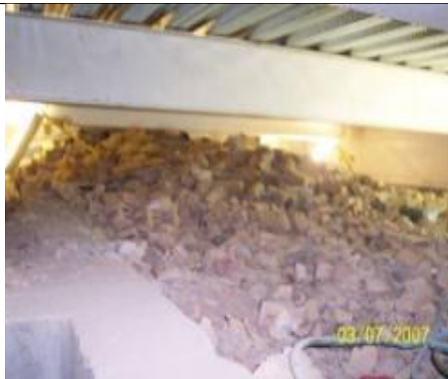
Rubble left in sub-floor void at end of construction project
