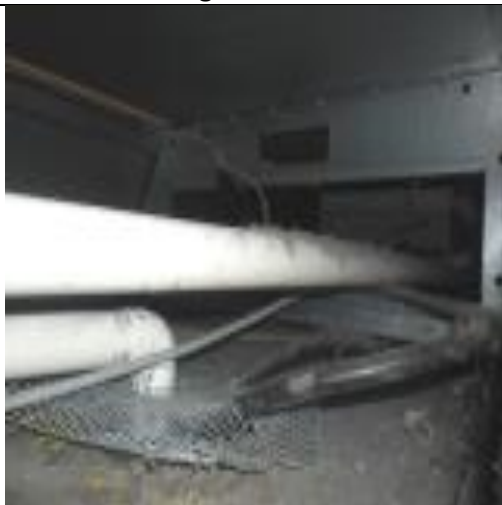
Services sealed with a metal cover plate
