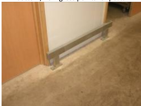
Wall protection barrier
