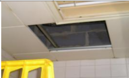
Ceiling tile which can be easily lifted to allow for monitoring and inspection
