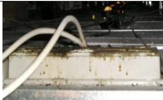
Heavily mouse smeared light fitting in false ceiling
