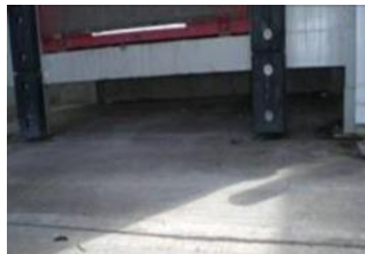
Gaps under dock levellers (tail lift slot) provide harbourage areas for pests and are a litter trap
