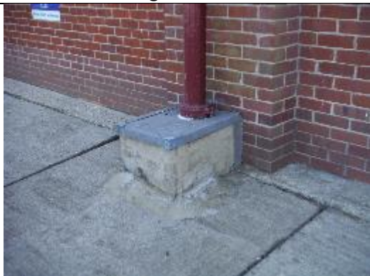
Storm-water drains are less prone to rat problems, but proofing further reduces the risk
