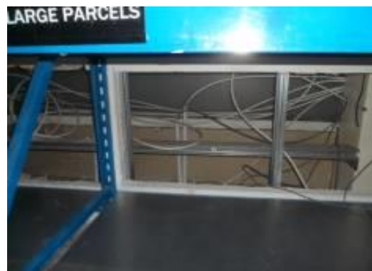
Cavity creating panels have had to be removed from this infested area in a retail storage area.
