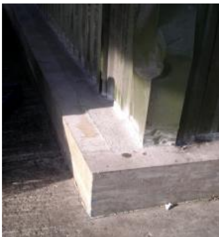
External cladding panels embedded in concrete; this should be sloped to shed water
