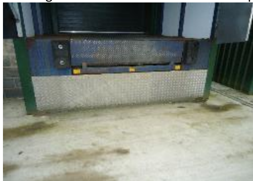
No gaps or voids in external walls or cladding around scissor lifts or dock levellers
