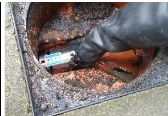
A purpose-designed rat blocker device being fitted into the sewer system
