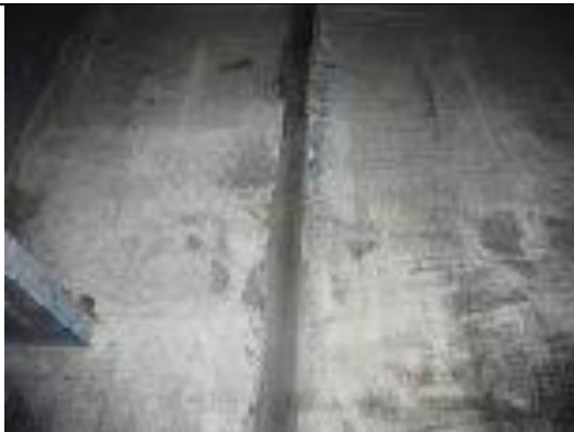
Effective expansion joint seal in a central area.
